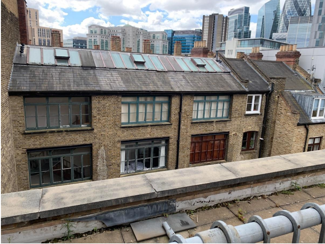
View from the existing roof terrace toward the former Soup Kitchen.
