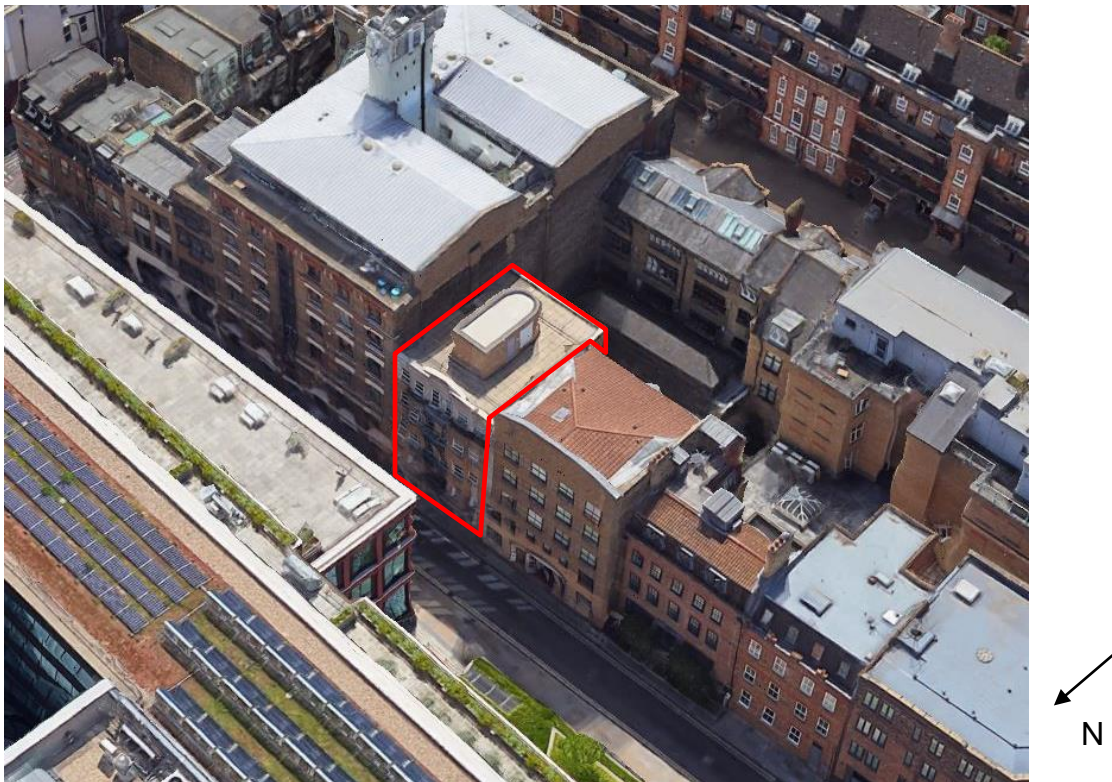
Figure 1 – Aerial photograph of the Site, view of the northern Whites Row elevation
